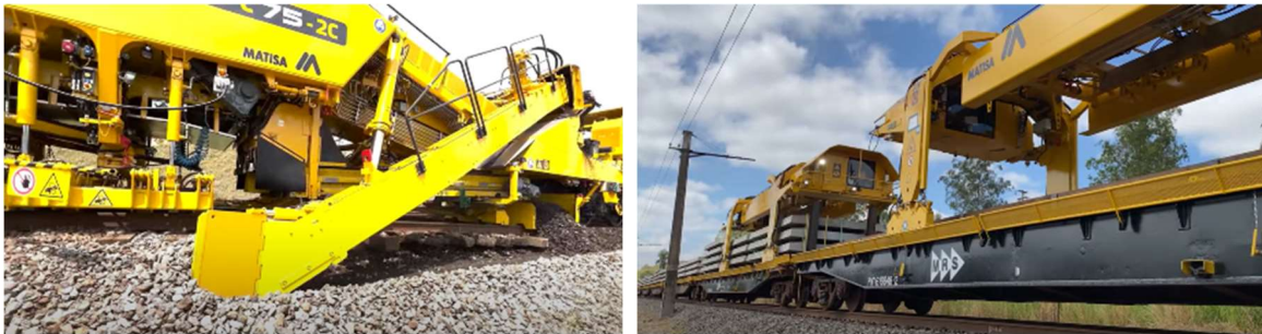
Figure 12: MRS ballast undercutter and track renewal machine in operation (Source: MRS)
