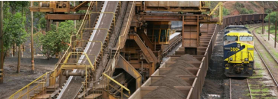
Figure 44: Silo loading terminal
