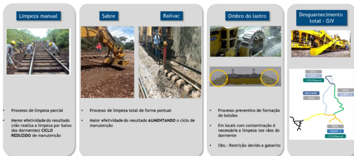
Figure 22: Ballast cleaning and recovery procedures
