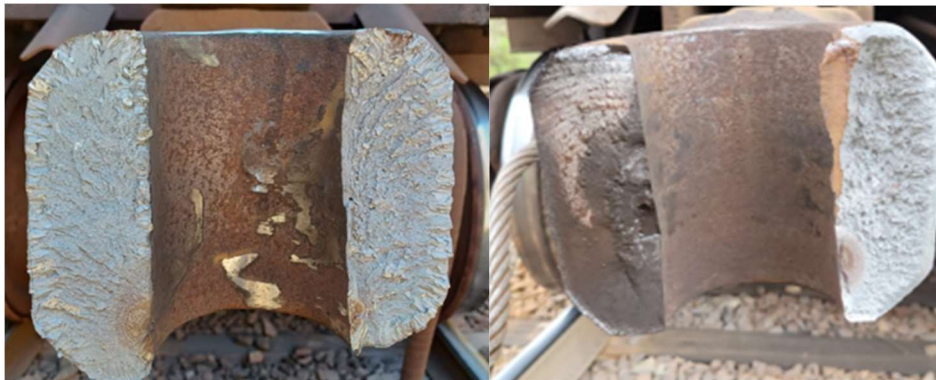
Figure 40: Fractures in the coupling system (Source: MRS)
