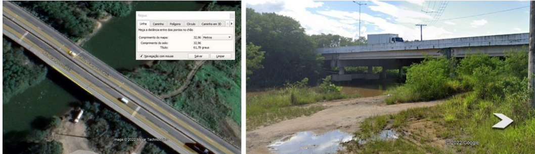
Figure 14: "Canal dos Escravos" bridge
