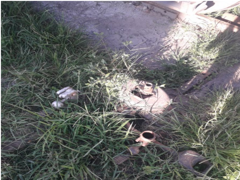
FIGURE 17 - LACK OF PROPER IDENTIFICATION AT DERAILER AREA
