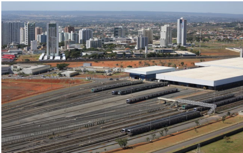
Figure 4 – Maintenance yard of Metrô-DF
