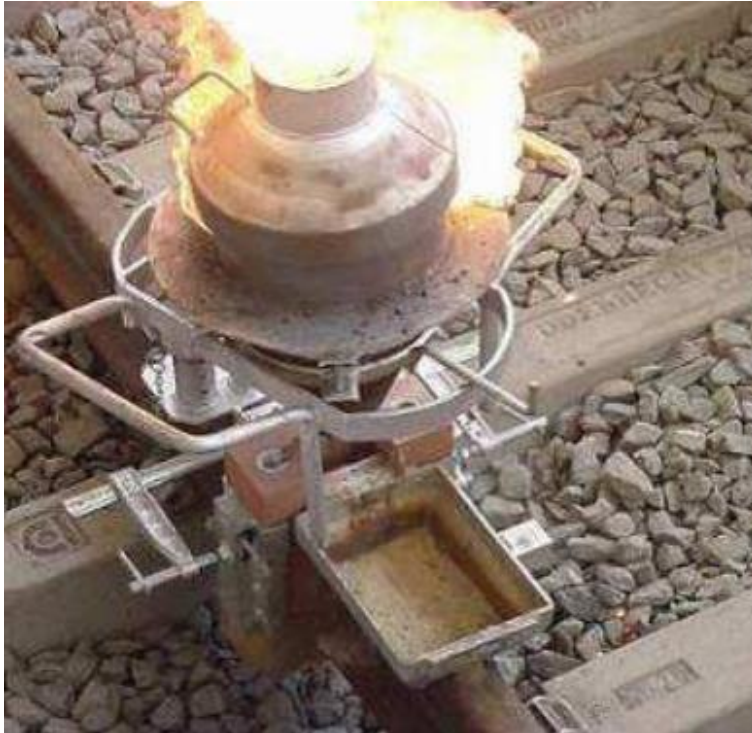
Figure 18 – Aluminothermic Welding. Source: MRS Logística
