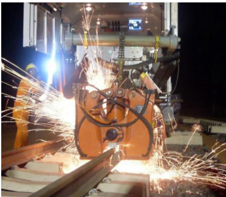
Figure 21 – Flash butt machine in action. Source: MRS Logistica
