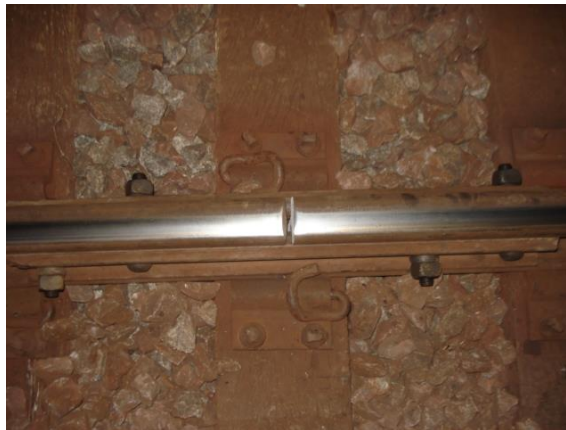
Figure 2 – Supported joint. Source: Authors
